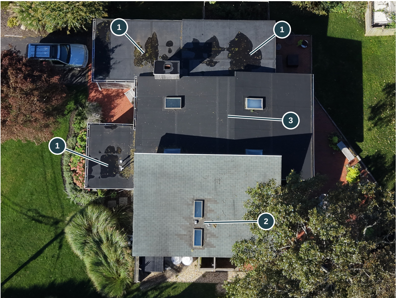
Overview from photo 0086. Marker 1 appears at three locations.
